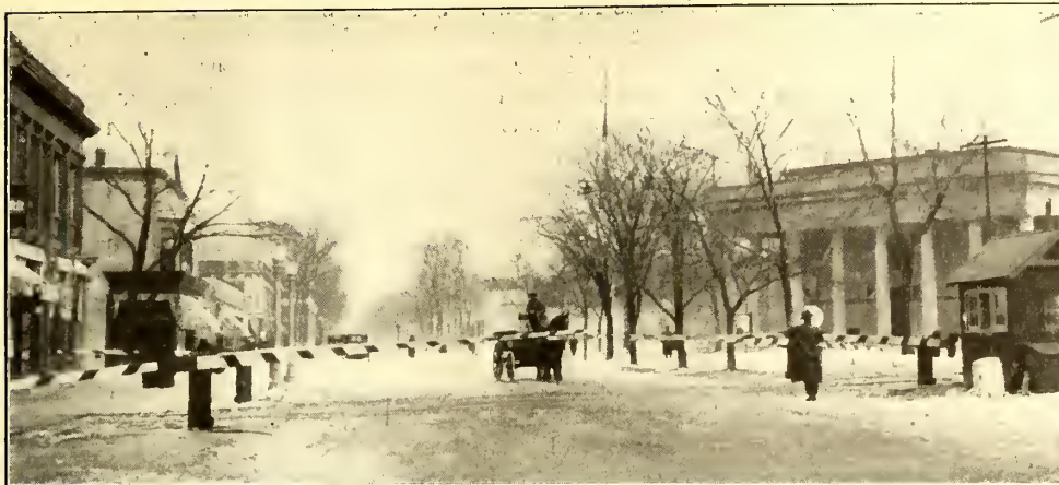
NORTH SHORE GRADE-CROSSING PROTECTION—CROSSING GATES PAINTED IN STRIPES TO ARREST ATTENTION; CONTACT DEVICE FOR WIG-WAG CROSSING SIGNALS
